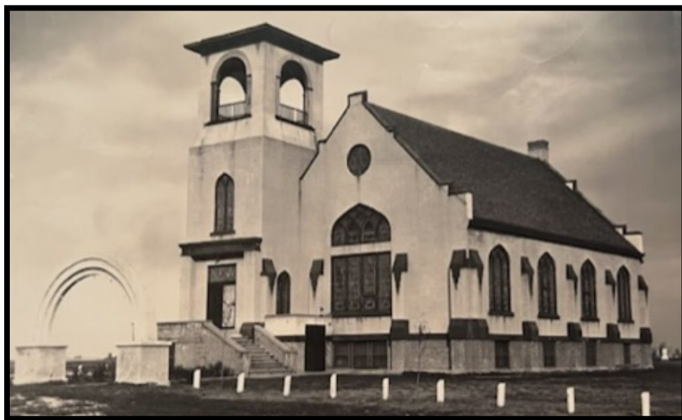
Bergen Lutheran Church rebuilt in 1921.
